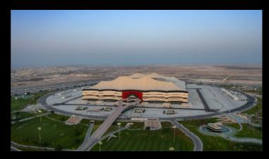
One of the big topics around the Qatar World Cup was the temperature. The Stadiums distinctive peaked shape is achieved with a polytetrafluoroethylene (PTFE) woven fibreglass membrane and with a retractable roof that complements the stadium's cooling technologies.
